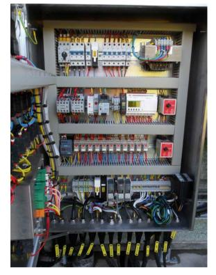
M&N's dedicated electrical control panel team fabricated a bespoke state-of-the-art unit to control all aspects of the MNSS5's functionality, including the modifications detailed by the technical team.
