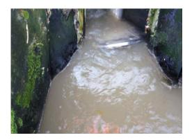
• Heavy flow to bypass channel further hampered by restrictive 6-inch concrete inlet channel infrastructure
