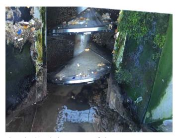
• Significant resultant backwash due to screen failure
