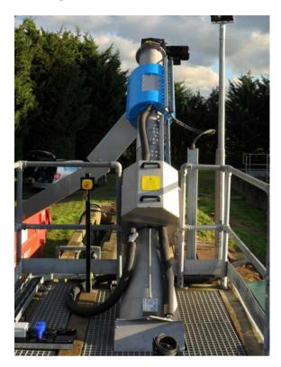
MNSS5 retro-fitted to existing STW infrastructure alongside new Control Panel with telemetry capabilities.
