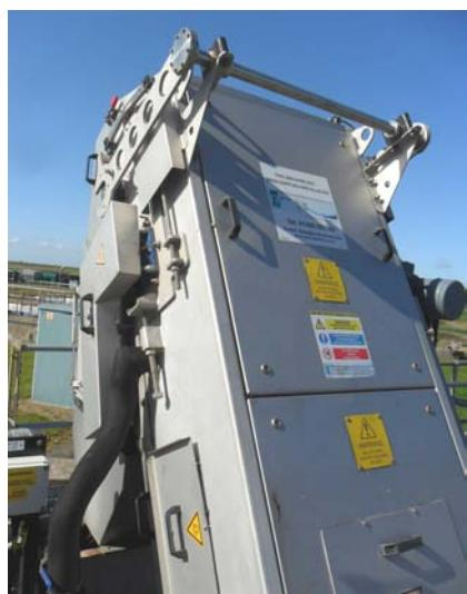
**A Frankenberger FSM Escalator Screen** was selected to meet both operational and budget targets. M&N's project team set about analysing site layout and existing infrastructure to develop a comprehensive installation sequence.
